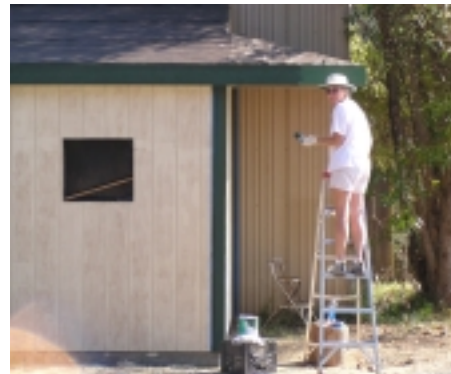
Painting the new addition
