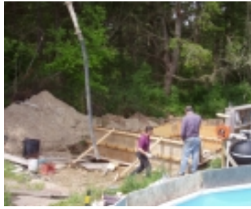
Pouring concrete for equip. shed
