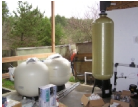
New filters and ozone contact chamber
