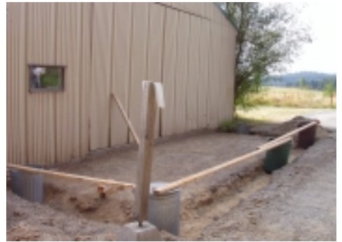
Foundations for addition
